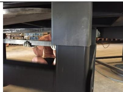
Align the standing support's verticals under the oven's standing feet with simple manual operations.
